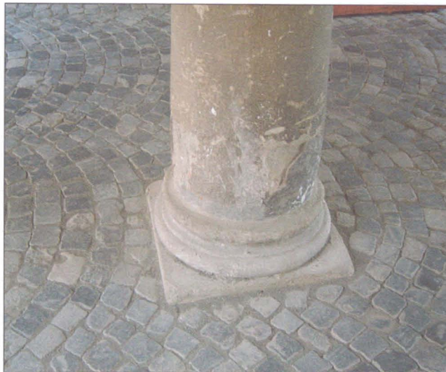
Figure 6. Servings socket on the left column presents the black crust of weathering of rock and parts of sulphates under attack from black crust. An important source of aggressive sulfates were introduced with Portland cement used in the finishing touches to the offsetting portions intense weathering - photo Drăgușanu.
