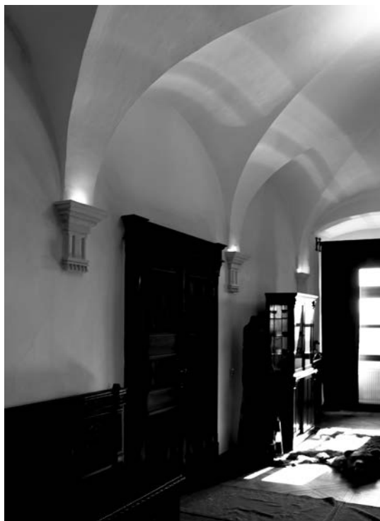
Fig. 6. Renaissance vaulting with corbels on the second floor (photo by László Pakó).
