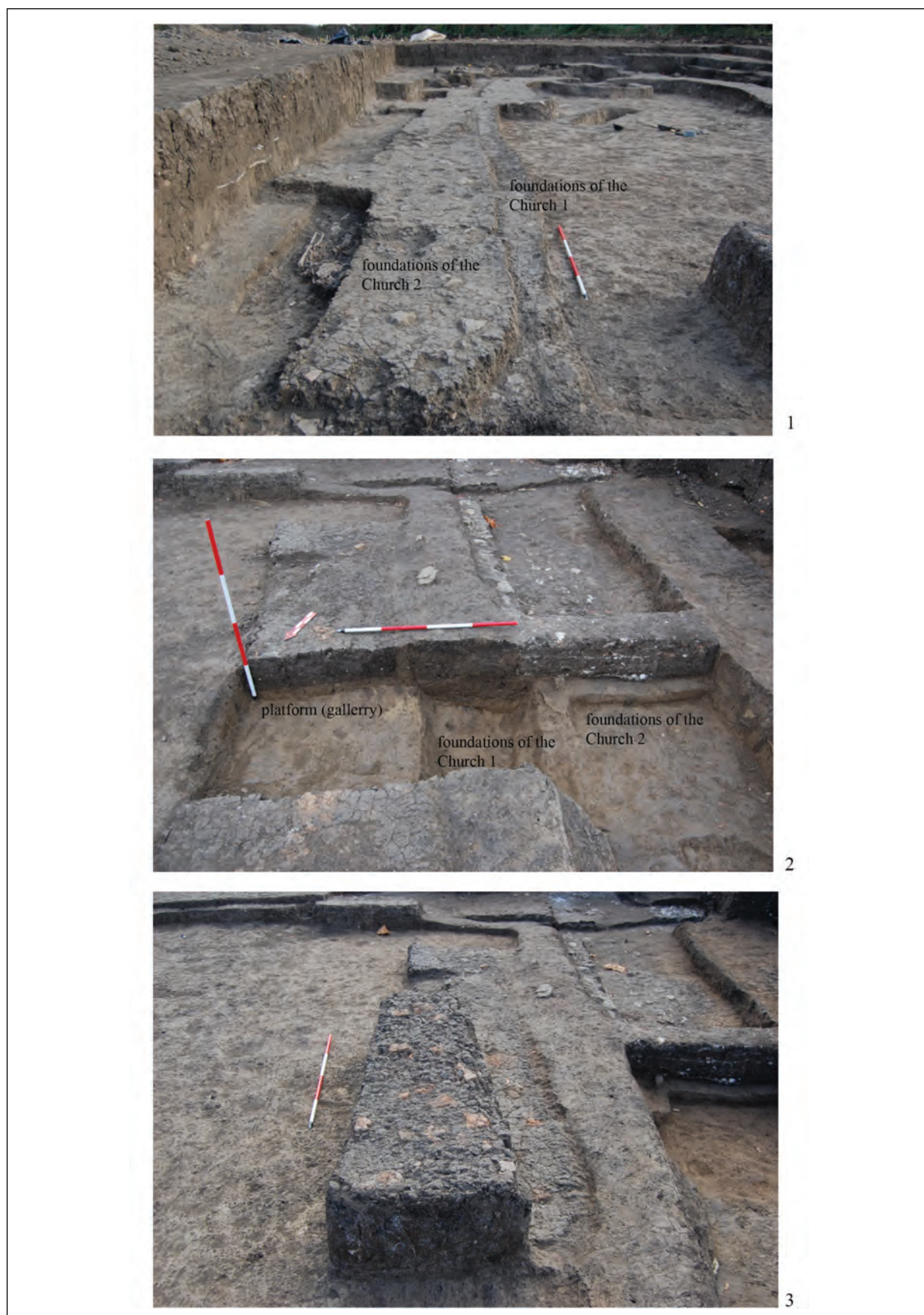
Plate 4. 1 – the relationship between the foundations of Church 2 and Church 1; 2 – cross-section through the foundations of Church 2, Church 1 and the platform in the western part of Church 1; view of the platform in Church 1 western part.
