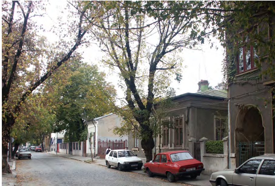
Fig. 5. Front of buildings that are not made by architects (Image of Plantelor Street).
