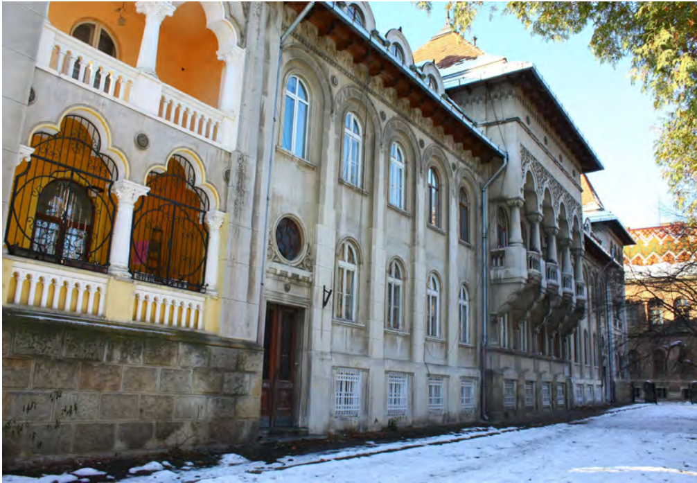
Fig. 3. Priests' House, 7 Kotsyubynskoho St.
