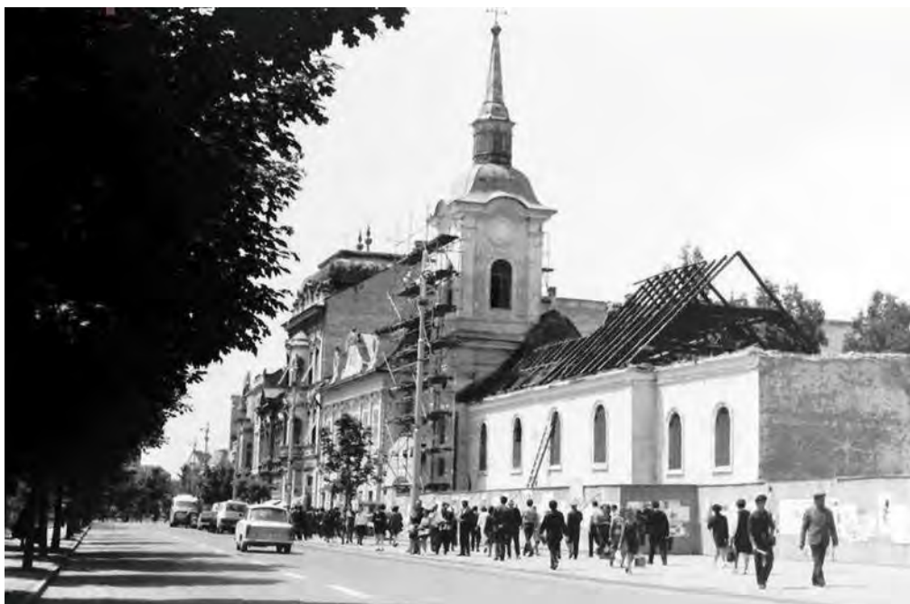
Fig. 8. The demolition of Franciscan Church.
