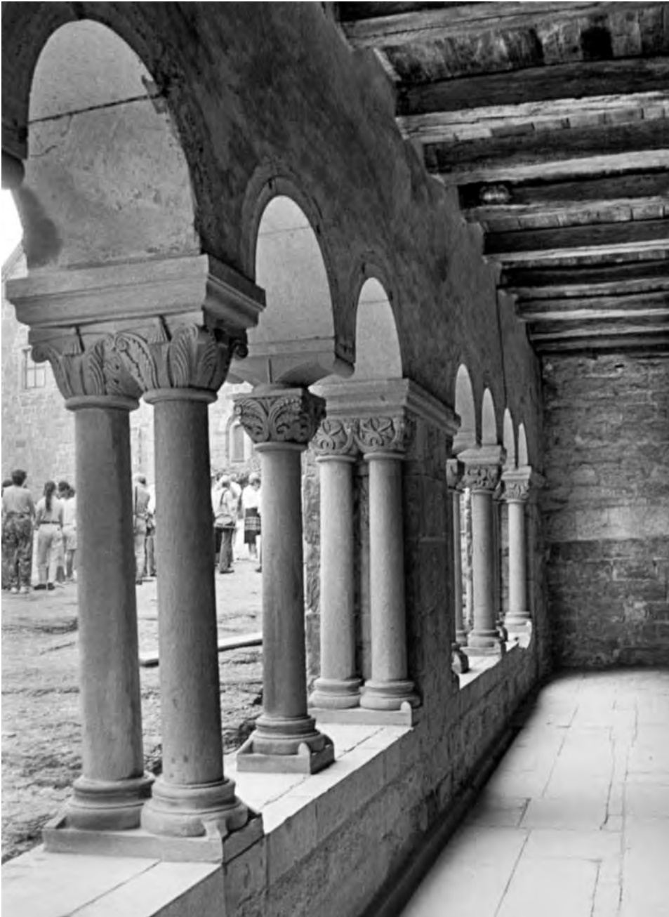
Fig. 16. Wartburg, near Eisenach (Thuringia), landgrave's dwelling, late 12th century: walkway.
