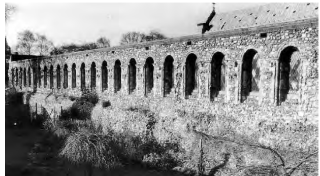
Fig. 11. Norwich Cathedral, 1096-c. 1140: north wall of the refectory (University of East Anglia).
