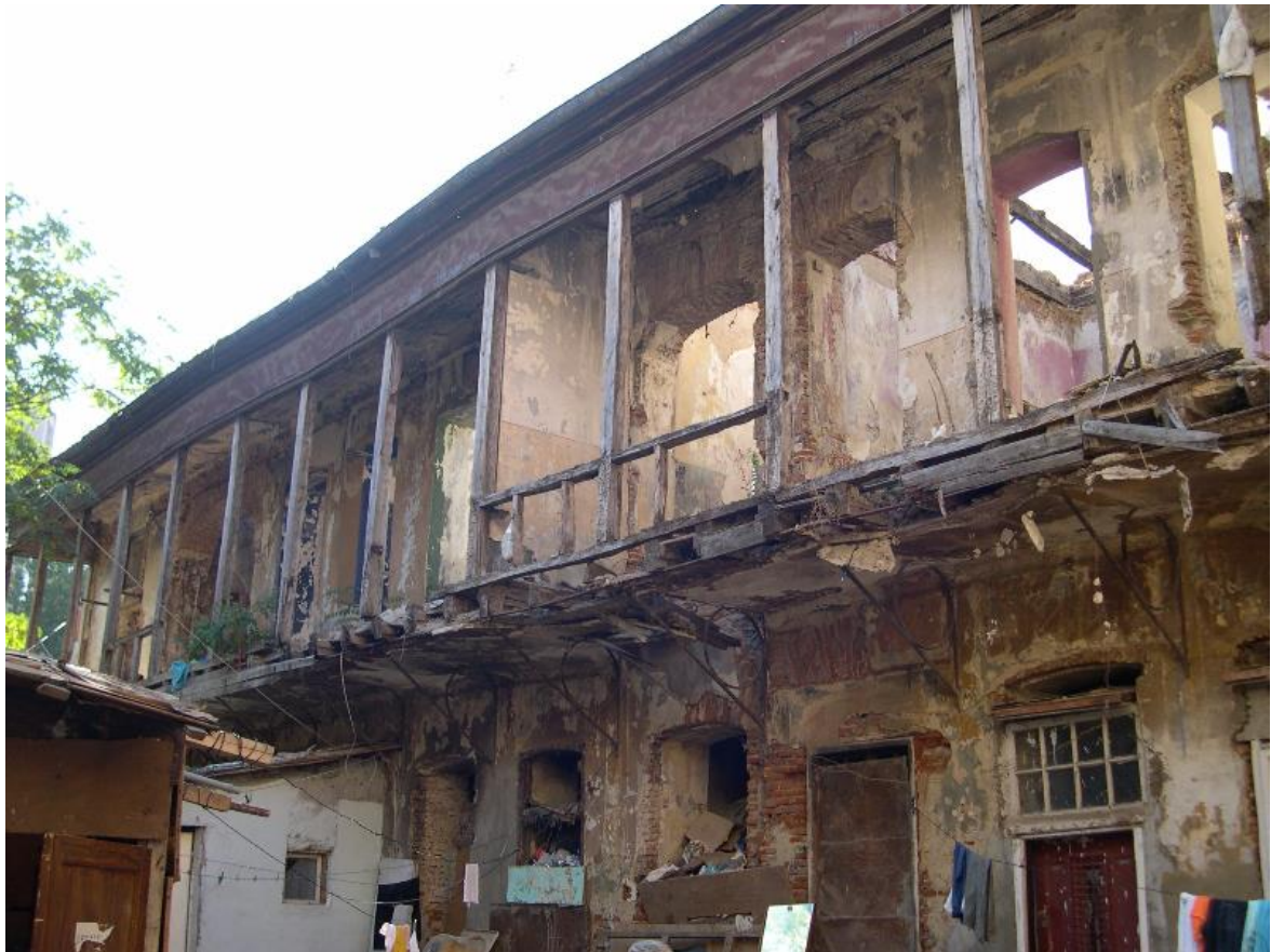
Fig. 11. Solacoglu Building. Image source: prof. Petre Mortu's archive.
