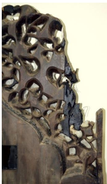
3. Losses of wooden material; detail
