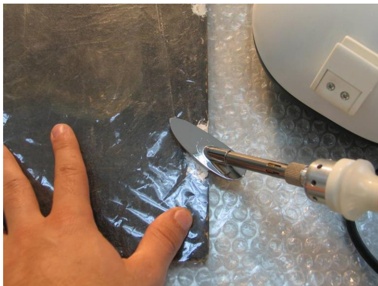
1. Filler levelling with heated spatula.
