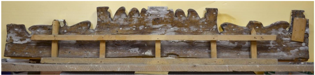
12. Decorative sustaining element; back view before restoration
