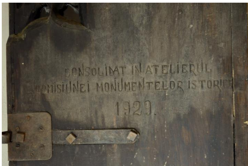
1. Dating inscription of the previous conservation and restoration intervention; detail
