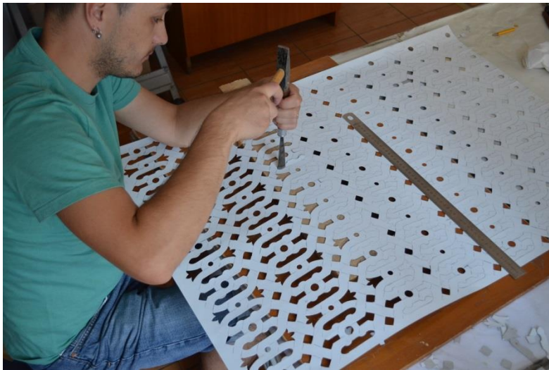
15. A cardboard template was made after the original background pattern
