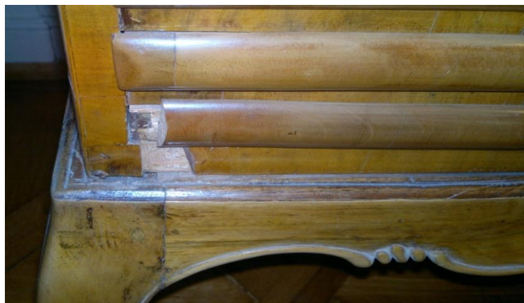
6. Detail; losses of wooden material
