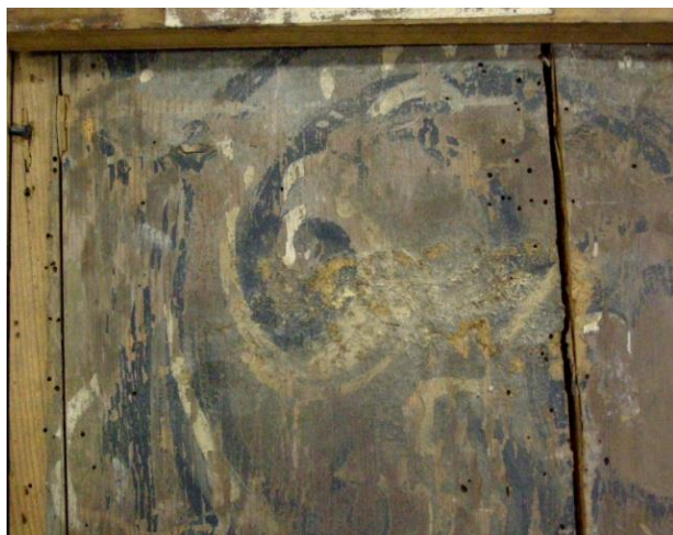
4. Detail; degradations due to the xylophages insects attack and the display system
