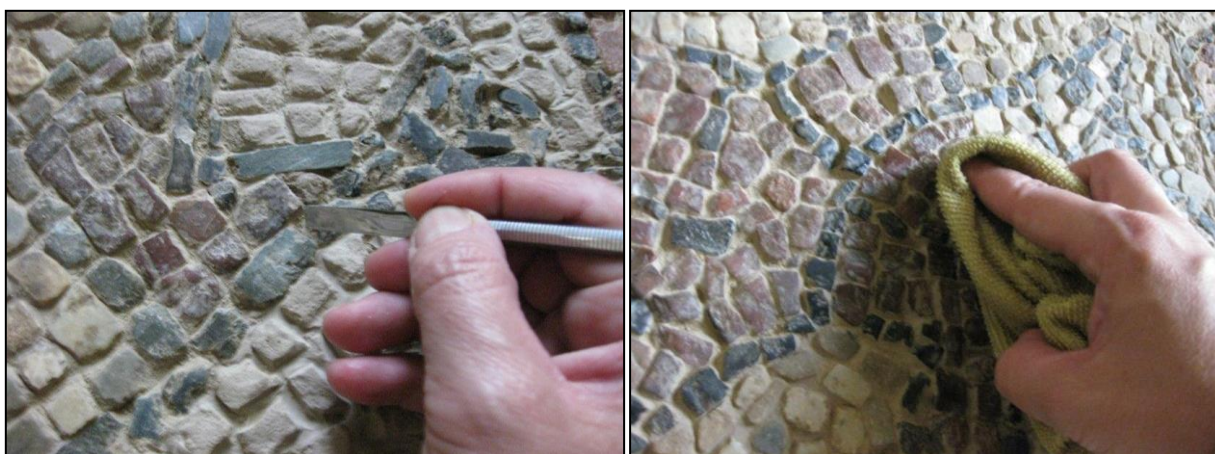
14 a, b: Cleaning the cement surplus and highlighting of the partings
