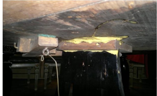
8. Detail; reattachment with polyurethane foam type adhesive
