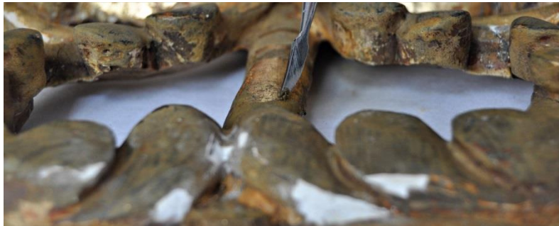
6. Detail – during removing of exterior primer
