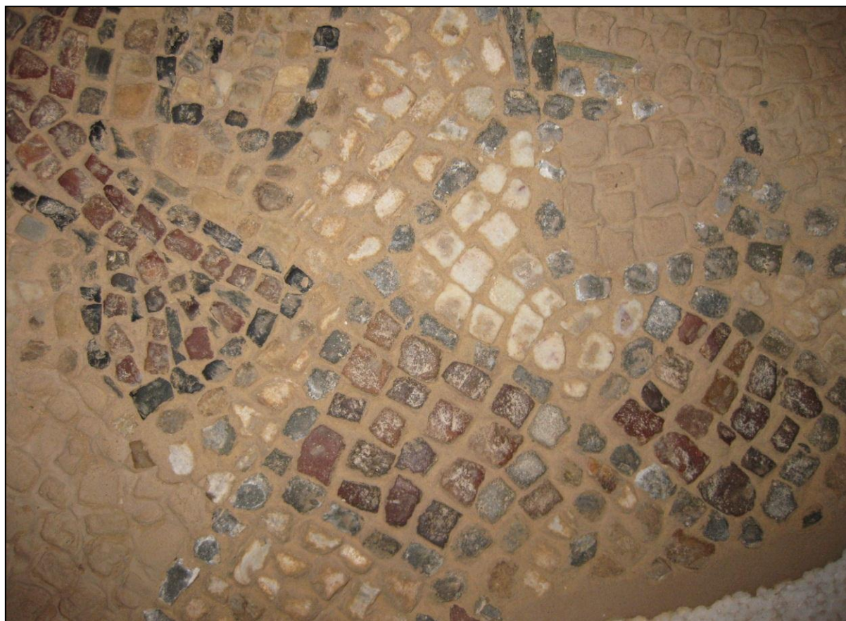
13. Details after the primary removal of the cement and plasticine surplus
