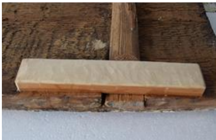
12. Details after restoration
