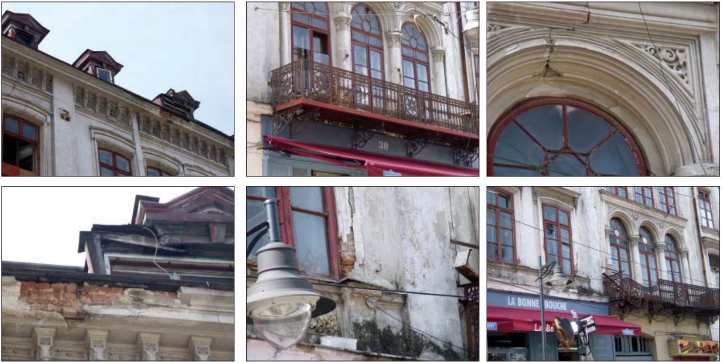
Fig. 20, 21, 22, 23, 24, 25, 26 - Tipuri de fracturi, unele extrem de periculoase
