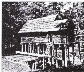
Water-mill with six horizontal wheels. Galesoala, Gorj County.
