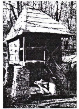
Water-mill with horizontal wheel. Toplet, Caras-Severin County.
