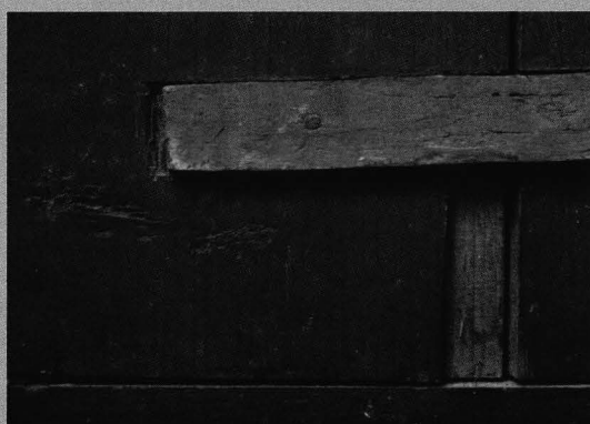
Fig. 8 Detaliu. Pierdere de material lemnos Detail. Loss of wooden material
