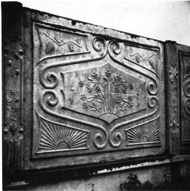
Fig. 20. — Prefabricated beton wall with « Modern Style » decoration — Cașin valley (Photo Paul Petrescu)
