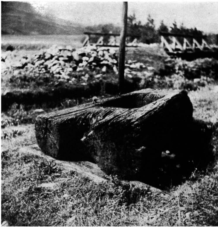
Fig. 13. — Wooden casing of a draw well — Brătoaia village (Photo Paul Petrescu)
