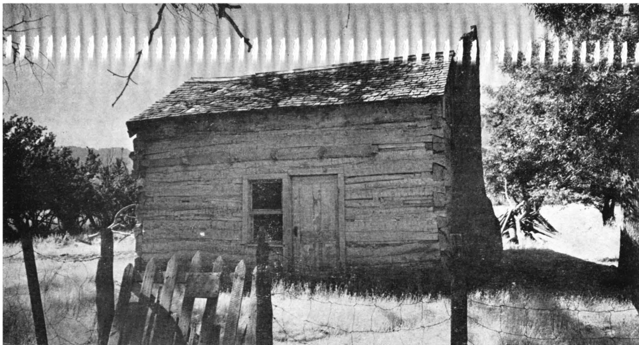
Fig. 14. — Log cabin, Grafton, with half-dovetail corners. (Photograph by Jan Brunvand)
