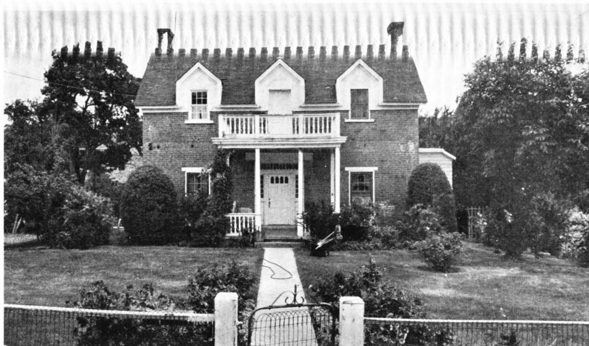
Fig. 23. — William Stirling house with Dixie dormers, Leeds. (Photograph by Jan Brunvand)
