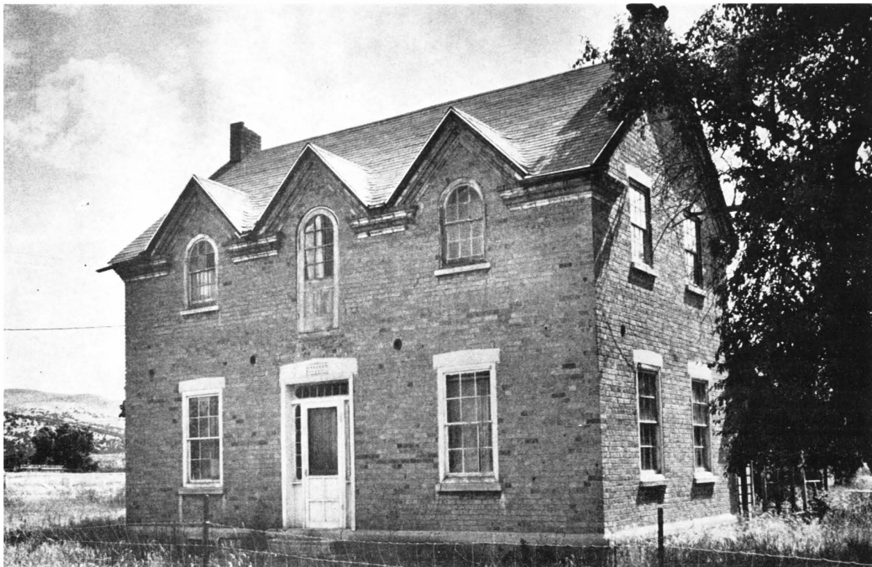
Fig. 13. — Brick house, Fountain Green. (Photograph by Jan Brunvand)
