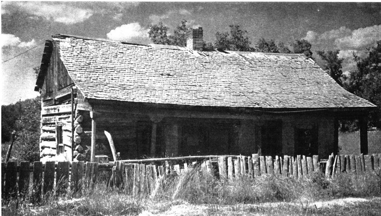
Fig. 28. — Log cabin with adobe addition at chimney-gable end and "Mormon fence", Spring City. (Photograph by Jan Brunvand)
