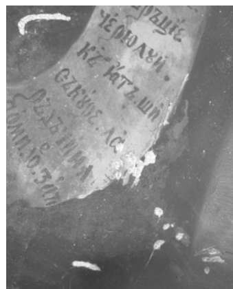
Fig.2 - Flight orifices on the surface of the painted layer
