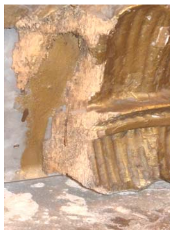
Fig.1 - Degradation of the woody support under the action of insects and fungi
