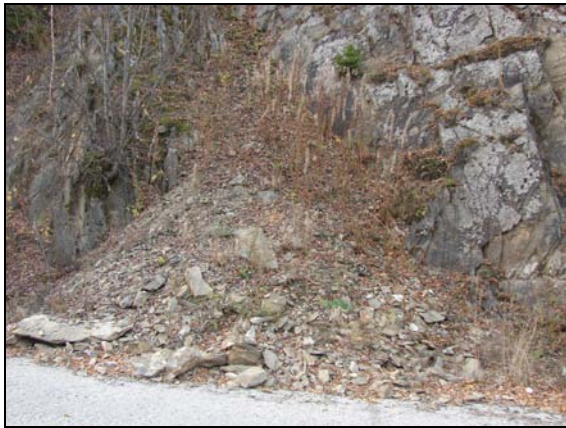
Foto 8. Debris cone with reinstalled vegetation
