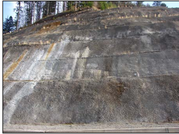
Foto 2. Right side of the embankment Gura Apei (reinforced)
