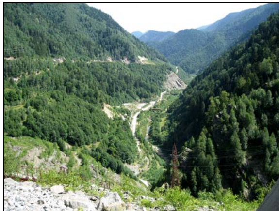
Foto 10. Downstream of embankment Gura Apei
