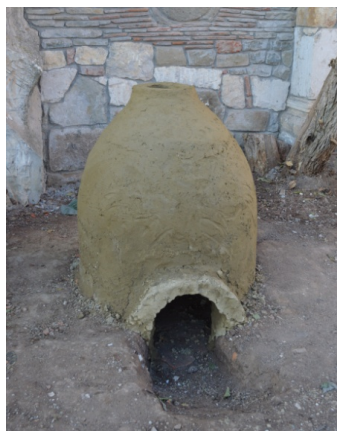
Figure 3.1–3.3. Different stages during the construction of the kiln.
