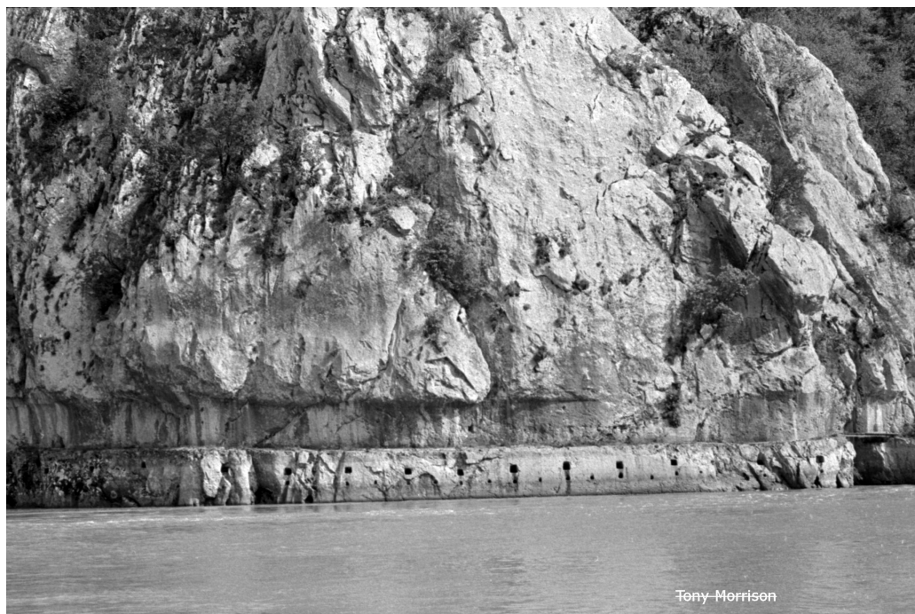
Figure 2. The photograph of the remains of the Roman road cut through the cliffs of the Iron Gates gorge, showing also the holes for the consoles. The photo is a courtesy of its author, Mr. Tony Morrison who took it in 1966
