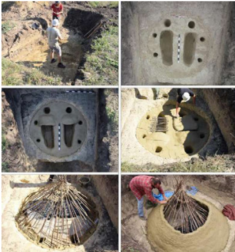
Fig.3. The experimental kiln – various stages of the construction
