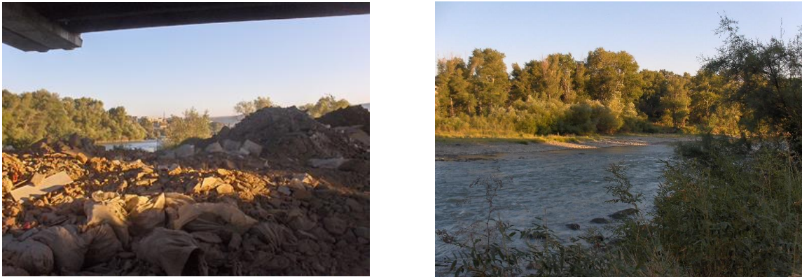
Fig. 4. Dighomi Floodplain today. Otter Island waiting for decisions on rehabilitation (Photos by G. Giorgadze, 2023).
