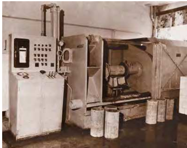
Interior resistance test
