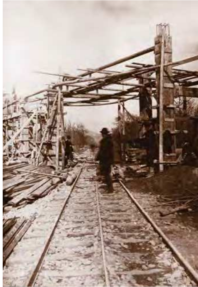
Conduit of the water channel constructed up until 1920, through which the waters of the lalomița River were conveyed to the I. M. Voith turbines
