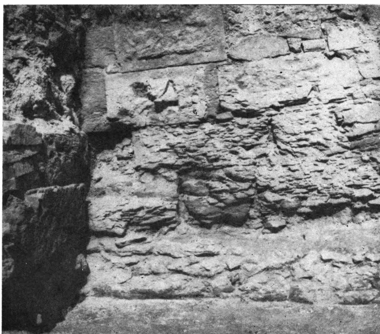
Fig. 14. Independența. S2 □ 4–6. The northern gate. The wall of the western tower.
