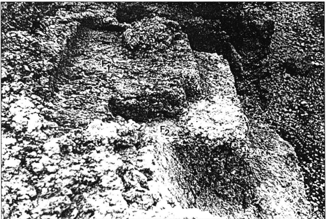
Fig. 8. View of part of a supposed foundation of anchorage facilities atop of the cliff fronting the Păcuil lui Soare Island. At about three meters above the water mark, the leveled rock surface shows various meter-size, shallow, rectangular cavities (F1), some open ended (F2), and small, deep vertical hollows, carved probably to support and anchor a wooden superstructure destined for ship loading along the cliff. In addition, broad, inclined skipways (T1), accurately incised at the sheer cliff edge, served probably for carrying wares down to ship decks.
