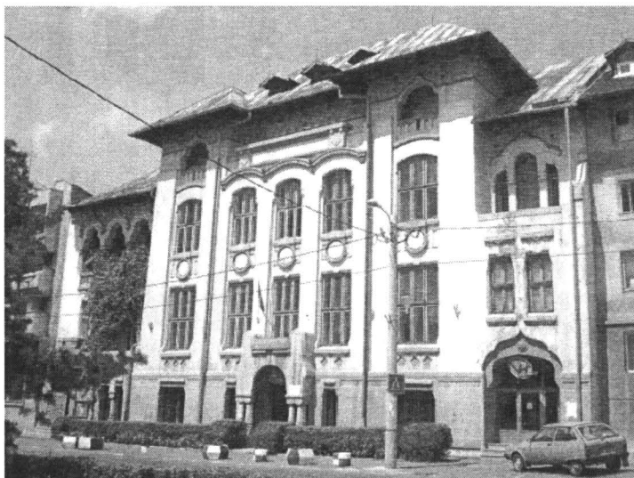
Fig. 1 The building of the Natural Sciences Department (Chimișliu, 2010)
