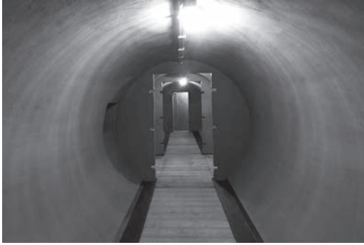
Fig. 8: Villa Torlonia, Mussolini's bunker, central corridor. Photo credit: Flaminia Bartolini.
