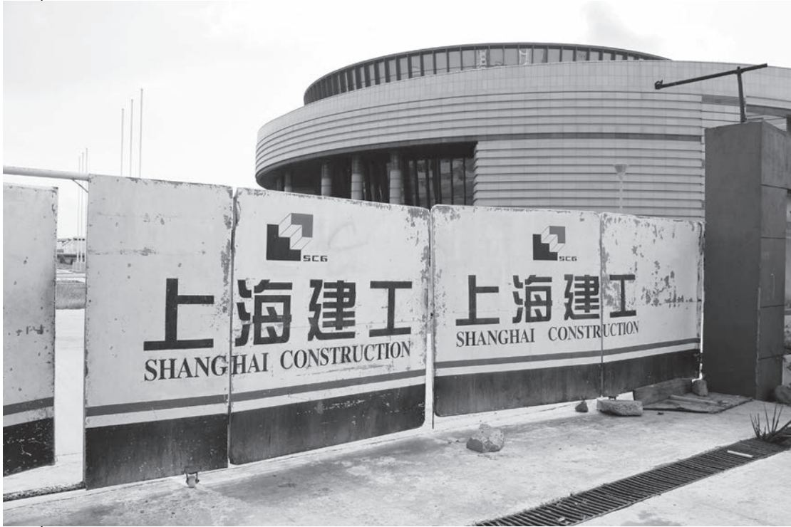
Photo 4: Construction Site of the MCN. Photo credit: Charline Kopf.
