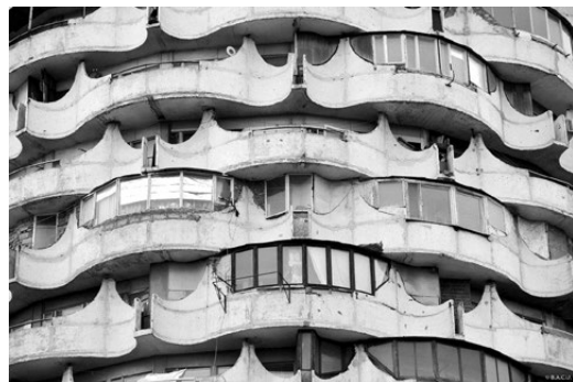
Photograph 1: Since 1990, the balconies of the building have been closed or altered in other ways by the residents. © B.A.C.U. photo department /2016.
