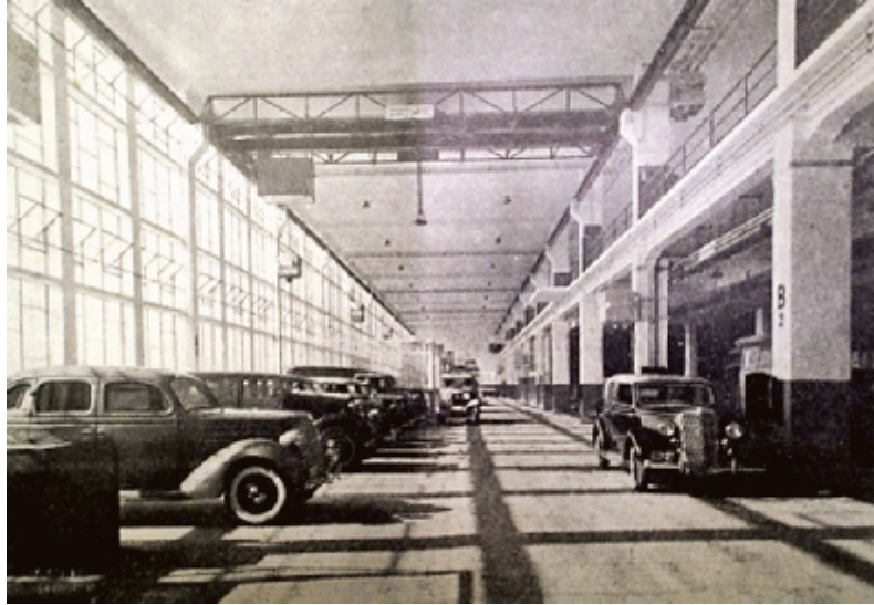
Fig. 5 Floreasca Assembly Plant – interior
