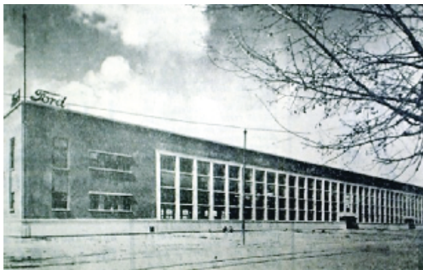
Fig. 3 Ford Assembly Plant
