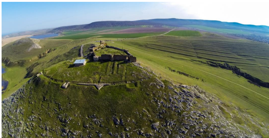
Fig. 2. Cetatea Enisala, fotografie aeriană dinspre nord / Enisala fortress, aerial photography from the north.
