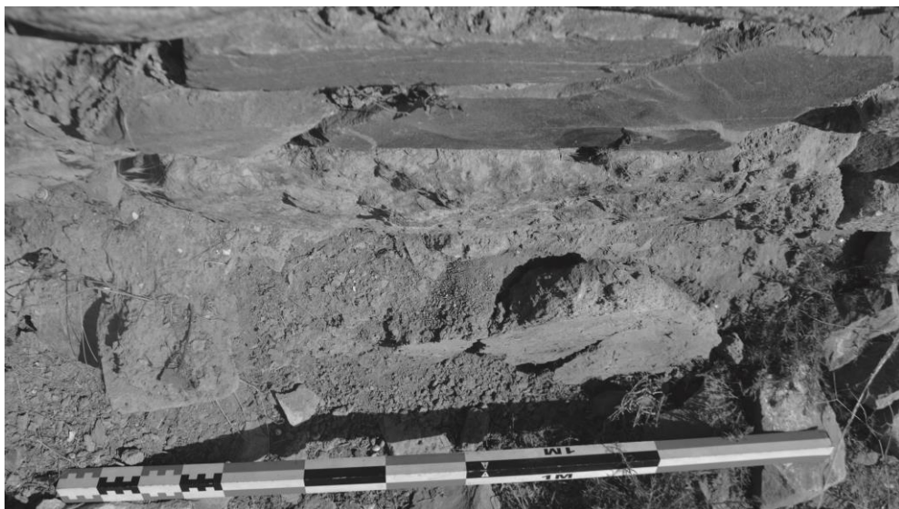
Fig. 28. Adobe insulation of the southern face of Z012 (V. Bottez).
