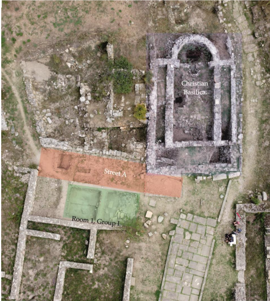
Fig. 1. "Basilica with Crypt" Sector and the surrounding area – drone view (photo: L. Cliante, 2022).
