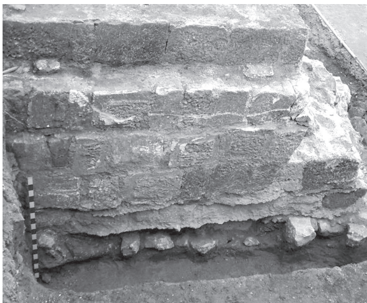
Fig. 6 - Section of the earlier fortress wall employed as a foundation for the 6 th c. fortification. Photo from the excavations of the eastern gates of Drastar.
