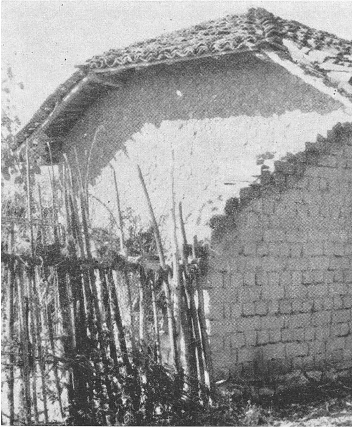
Fig. 7. — House made of adobe with brick fragments into the plastering (beginning of XX th century).
