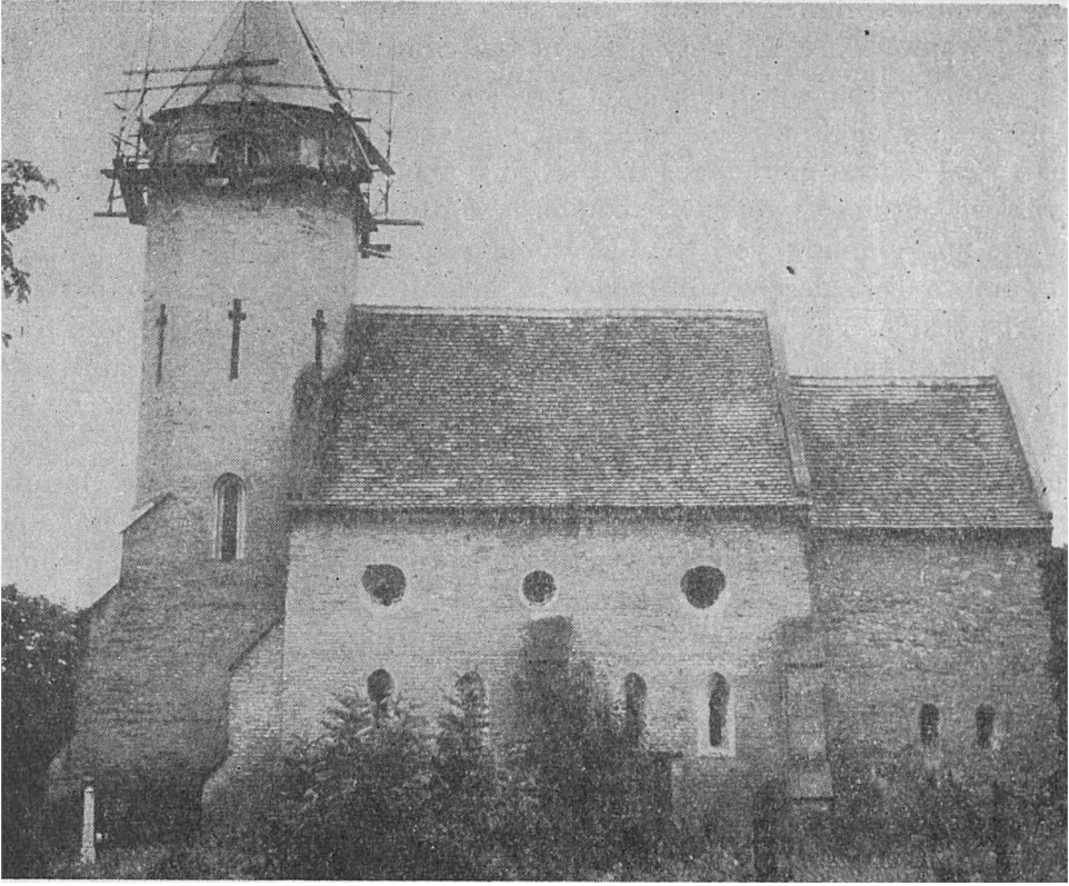
Fig. 7. — Morović, church of Sv. Marija, general view from the south.
