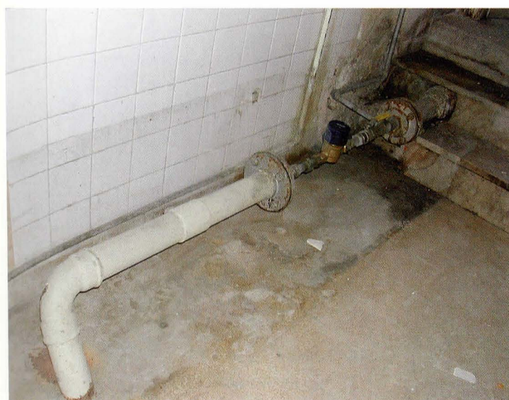
Fig. 14. Water supply pipes with leaks
