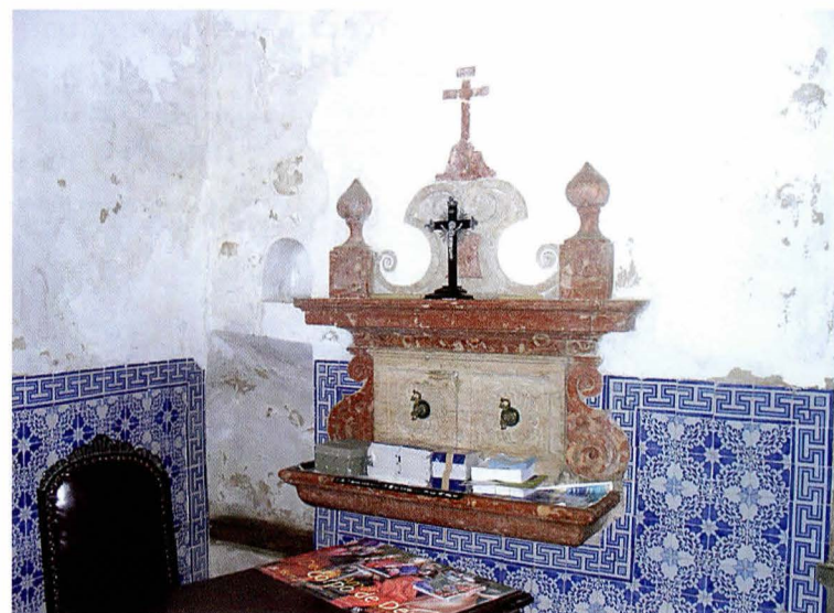
Fig. 15. Effect of condensation water
