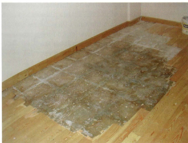
Fig. 2. Damage floor due to humidity
