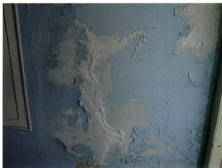
Fig.10. Salt migration for exterior
