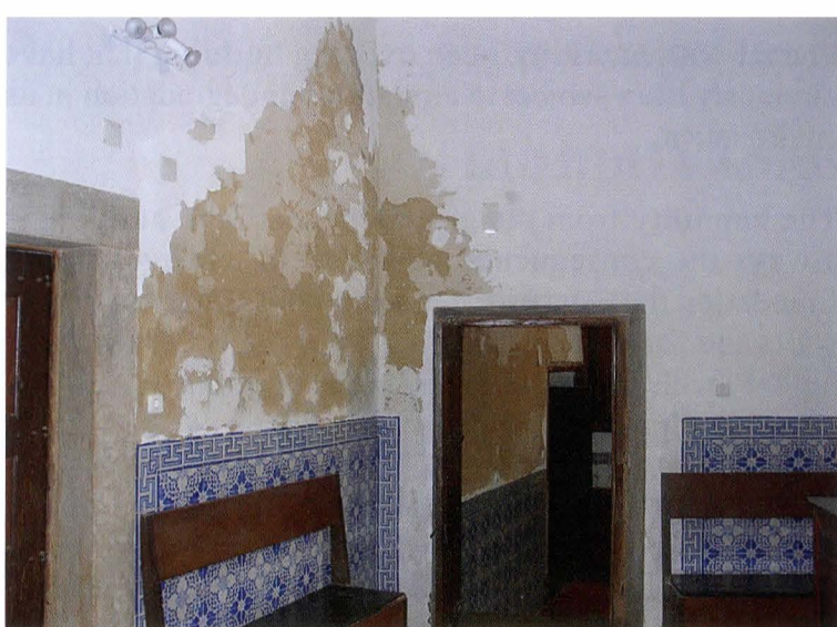
Fig. 5. Damages due to ground humidity
