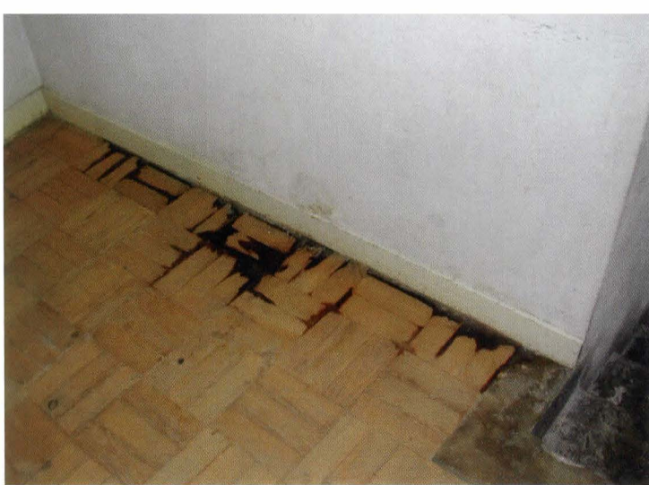
Fig. 1. Humidity in floor
