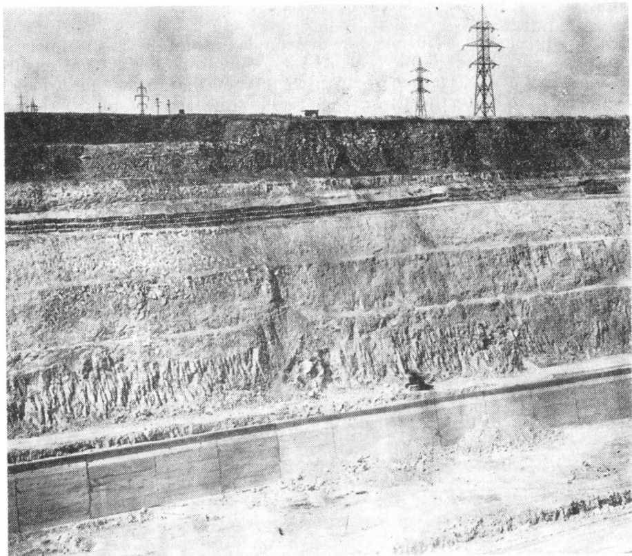
Fig. 1. — View of the canal section in construction (photo L. Căplescu).
