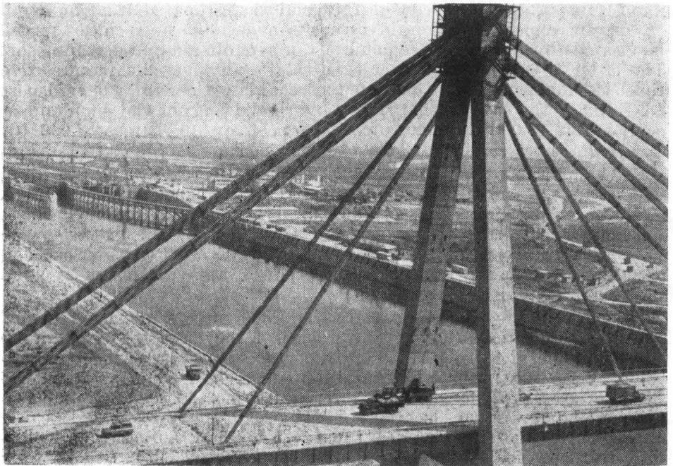
Fig. 6. -- The Agigea roadway bridge over the canal (photo Agerpres).
