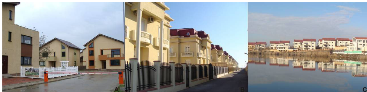
Fig. 8 – Residential development in the Bucharest Metropolitan Area (A – gated community in Corbeanca; B and C – residential projects in Voluntari).
