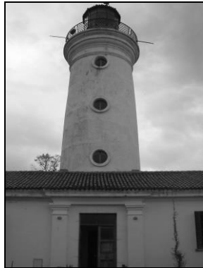
Photo 2 – The old lighthouse.
