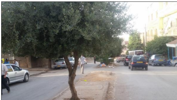
Fig. 8 – Sub-arterial road interrupted (Djebbar, July 2018).
