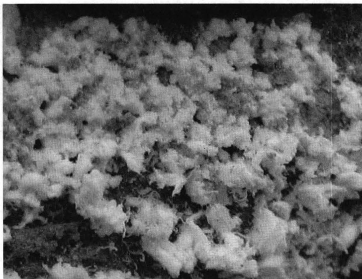
Fig. 4: Salts accumulation on limestone and cement on the footing of the church
