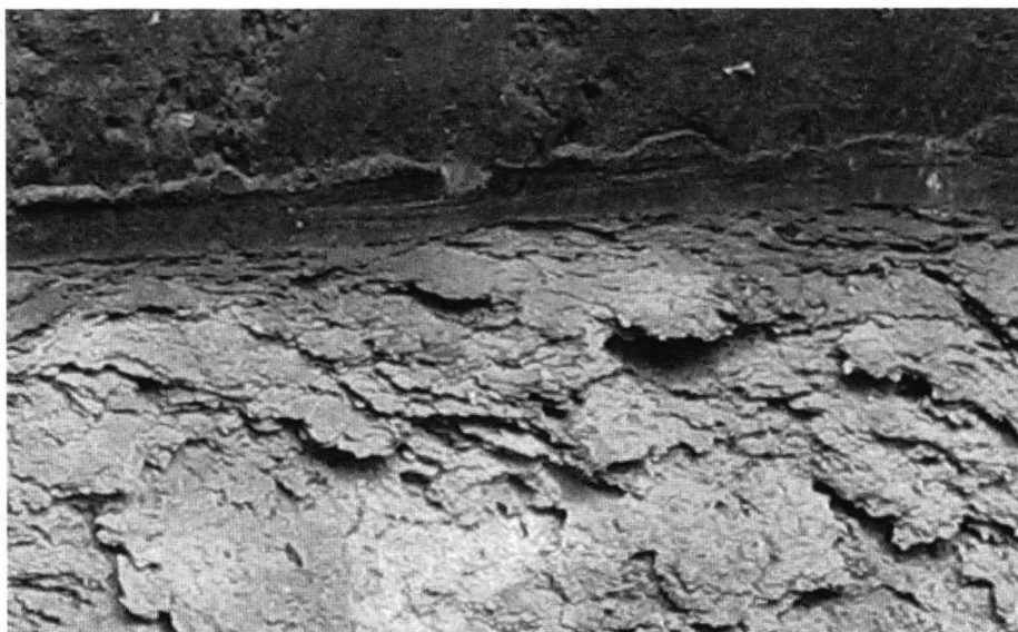
Fig. 5: The presence of the Portland cement generates the forming of the black crust. Under the cement's level the \text{SO}_2 anions attacked the limestone that is degrading by simple multiple and flake exfoliation.
