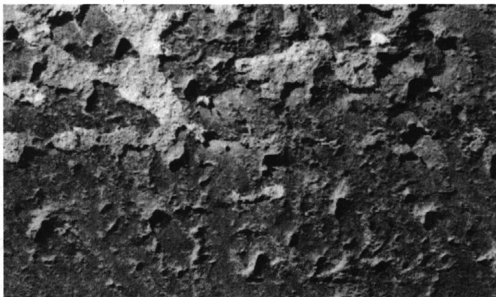
Fig. 1: Black sulphuric crust on the Baciulimestone that is exfoliating due to the different dilations on the surface, and because of the crystallization pressures of the sulphates and sulphides in the crust.
